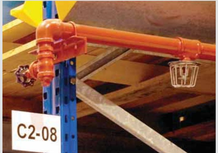
Sprinkler heads may be located within the racking, or in the gap between 2 sides of double faced rackings
