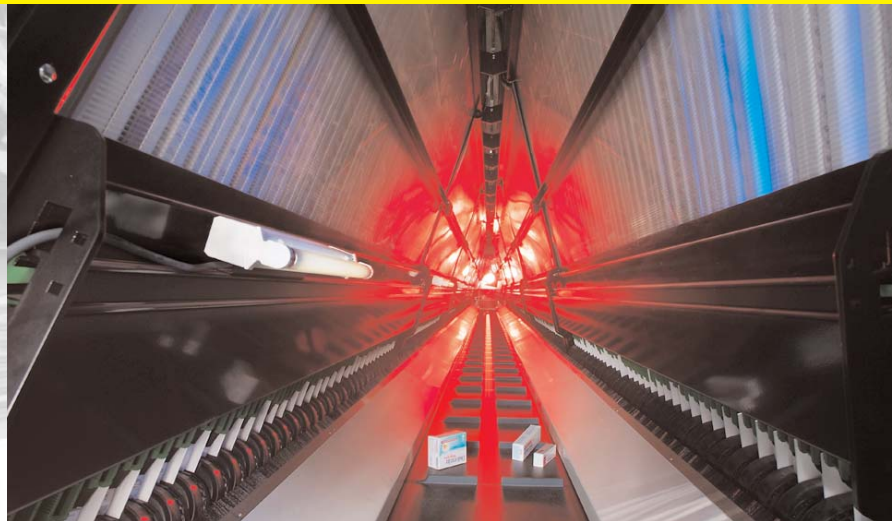
S-Pemat viewed from the inside
