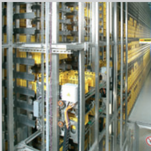
Raw materials warehouse with hoist
