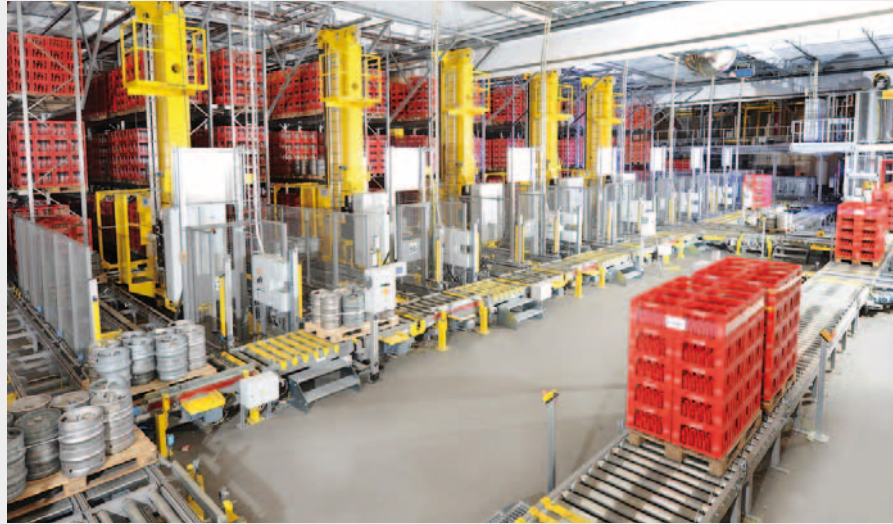
Buffer for empties with new SCC
