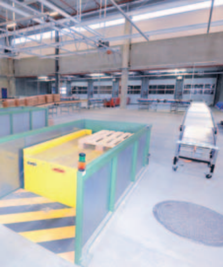
Vacuum lifter, hydraulic scissor type lift tables, roller and telescopic conveyors are the equipment for ergonomically designed work stations in goods receiving
