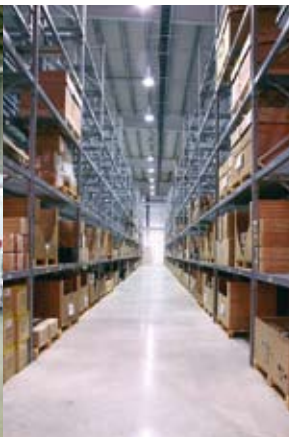
Shelf supported mezzanine construction in the BMW small parts warehouse in Incheon, Korea.
